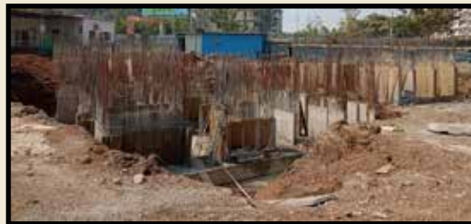
Dudulgaon A : Building Foundation and Plinth Work in Progress
