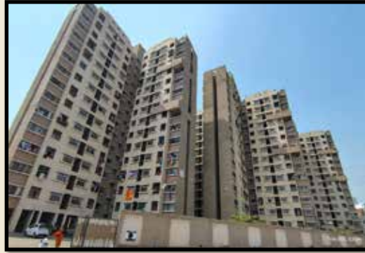
Charholi Project : 1,442 Houses (Till date Expenditure Rs. 169.43 Cr) Project Completed : July 2024
