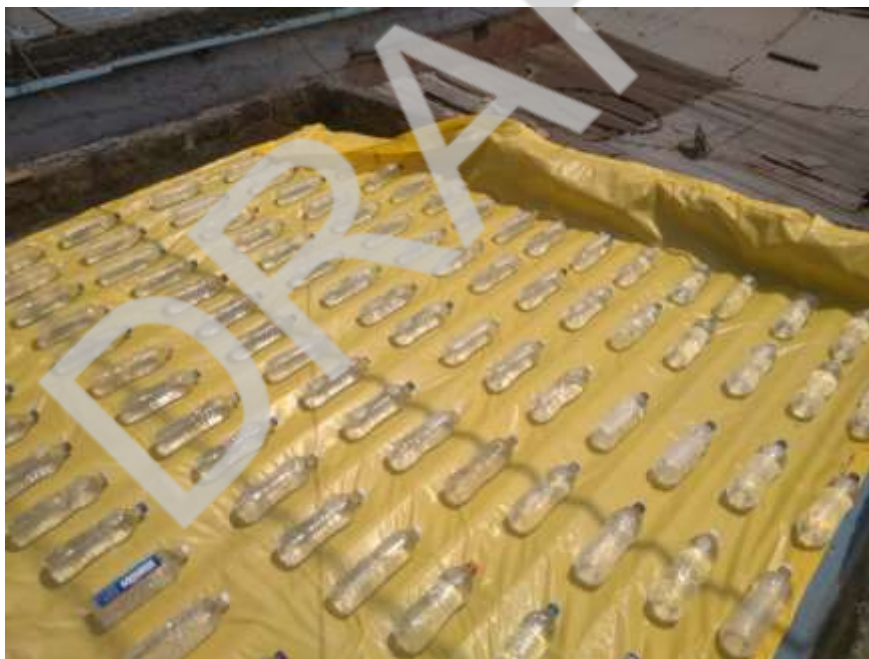
Figure 40 Water-filled PET bottles on a tin-roof
