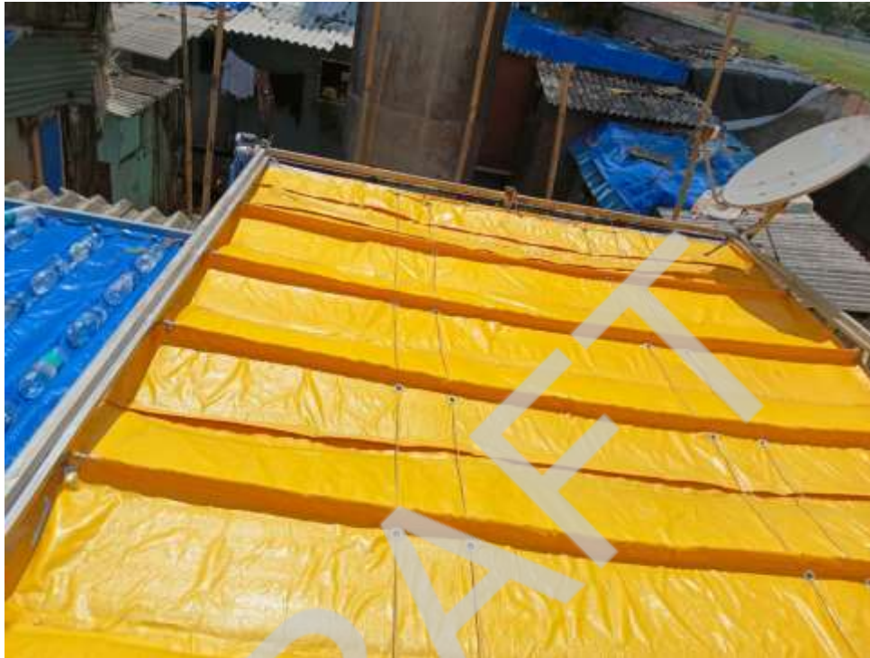
Figure 42: Alufoil Pipe Motor (on a tin-roofed house)
