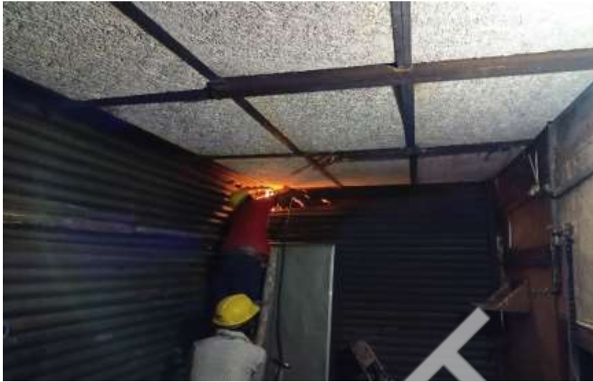
Figure 45: Wood Wool Panel (under a tin-roof)
