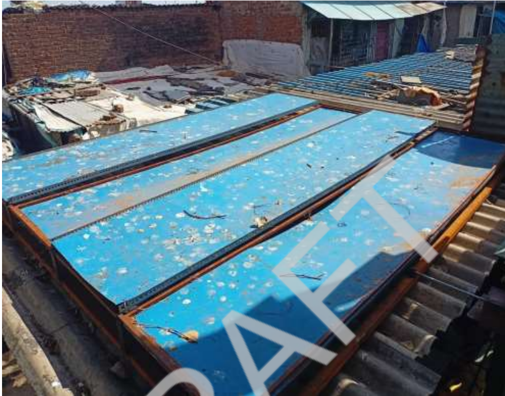
Figure 44: Alufoil Sliding (on a tin-roofed house)
