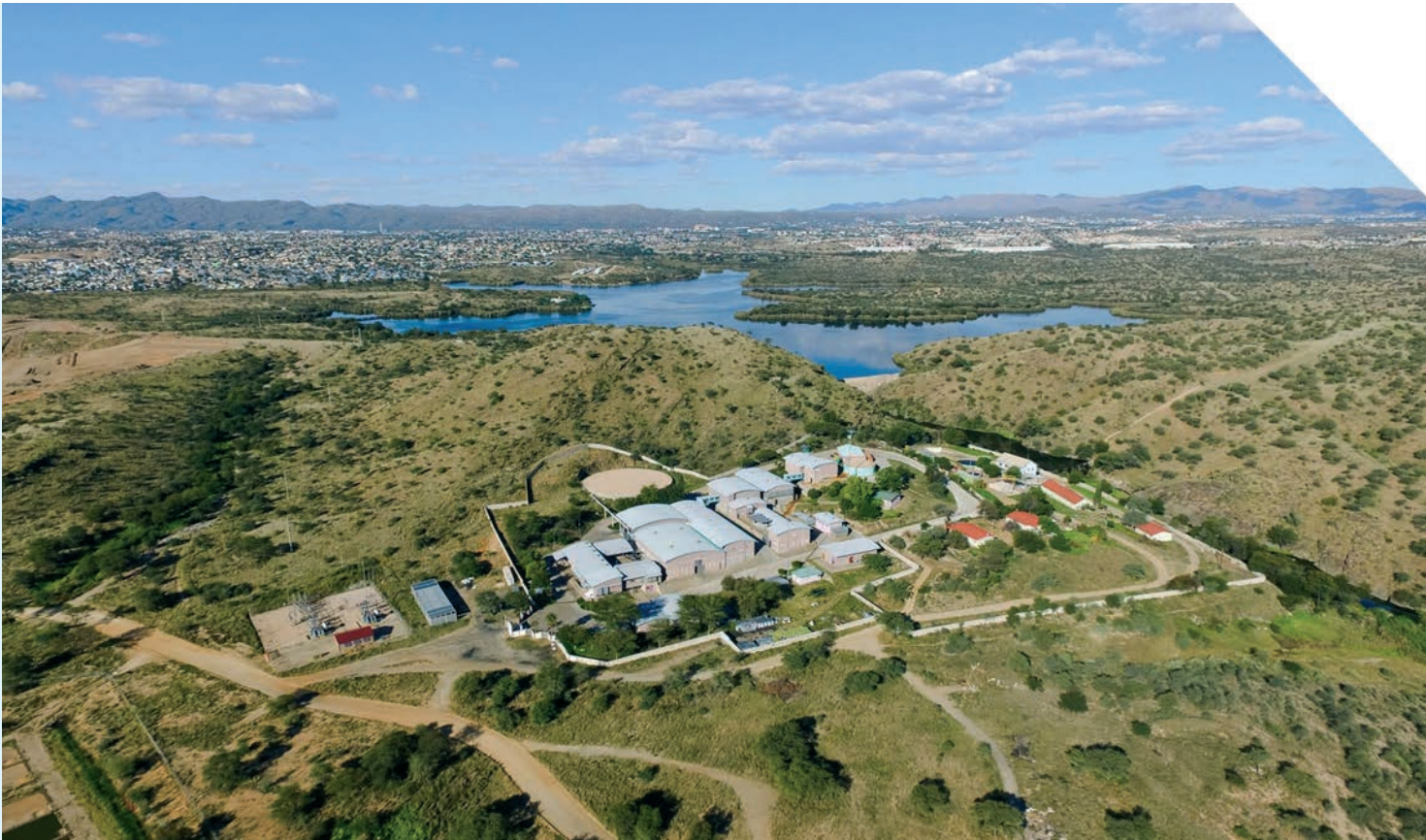
The Goreangab water treatment plant in Namibia uses a process that mimics nature to transform wastewater into drinking water.
